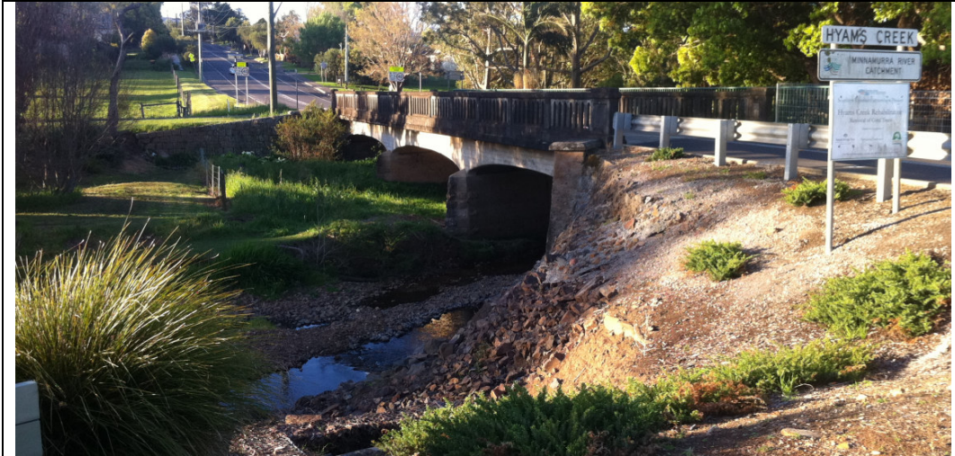
Figure 9. Hyams Creek bridge viewed looking toward the north (Albion Park)
