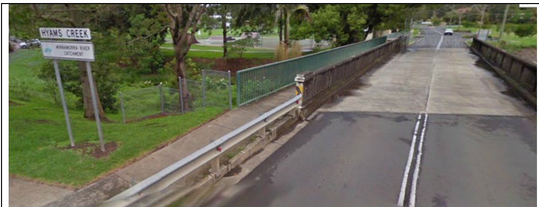
Figure 10. Hyams Creek bridge viewed looking toward the south (Jamberoo)
